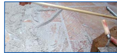
Grouting with epoxy resin-based pavement jointing.
