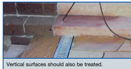
Apply Lithofin STAINSTOP ›W‹ with a spraying device.
